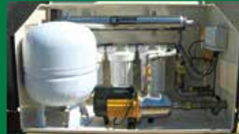
Rain Water Harvesting System;
